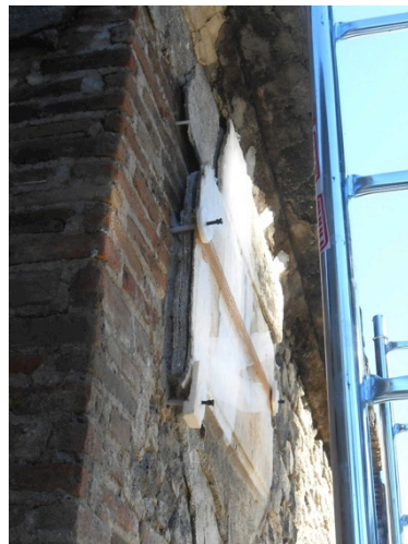
Three moments of the emergency interventions to secure very badly detached parts of the decoration.
