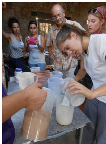
Preparing the foam and adding the hydraulic lime mixture to create the hydraulic foam to be injected in the detachments of the plasters.
