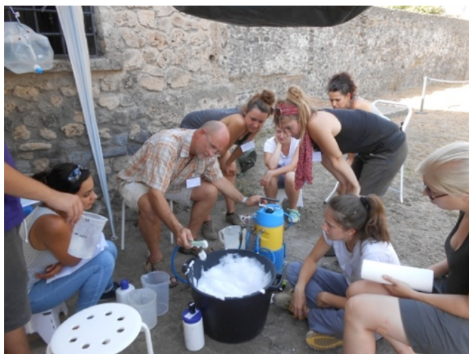
Preparing the foam and adding the hydraulic lime mixture to create the hydraulic foam to be injected in the detachments of the plasters.
