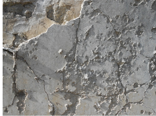
The damage of the surface of the stucco plasters, due to salt crystallization.
