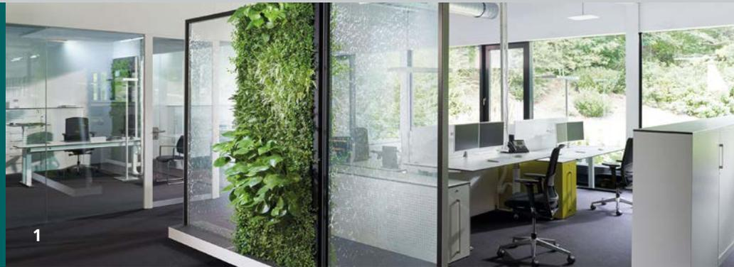
1 Comfortable air conditioning and effective indoor air dehumidification using the Chilled Water Wall, in this case placed in an open-plan office in conjunction with a green wall.
