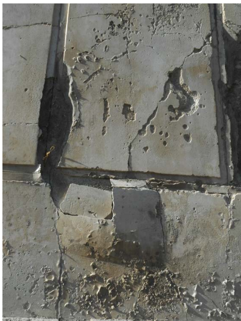
Fig 181 - Tomb 14EN, detachment of the final stucco layer + the 2nd preparatory mortar layer
