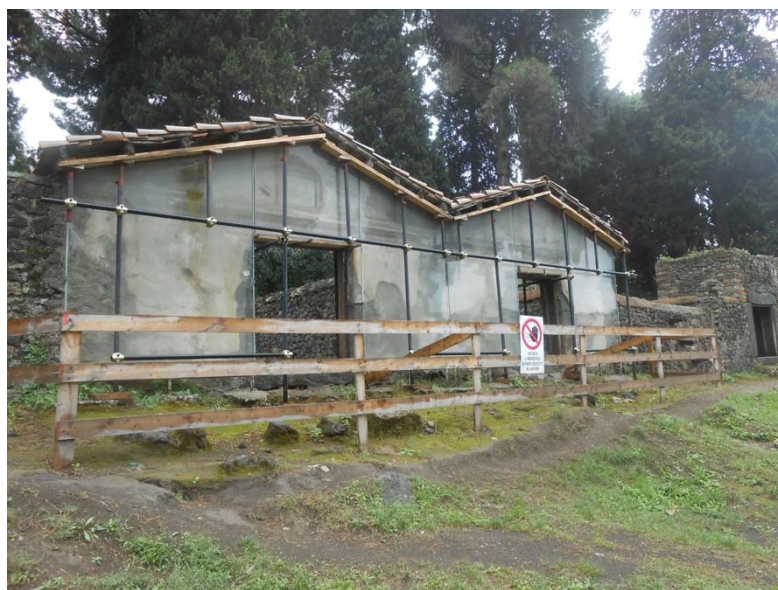
Fig 108 - Tombs 9ES and 11Es with modern propping of the tiles' roofs.
