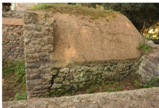
Figure 178: map 07_ES_W_I of delamination (detachment) from structure.
