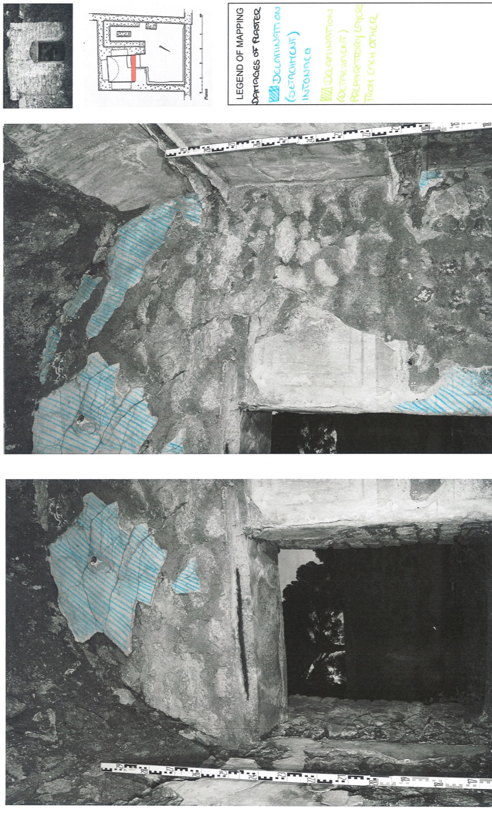
Figure 180: map 07_ES_N_I_2 of delamination (detachment) Intonaco from preparatory layers (blue) and delamination (detachment) preparatory layers from each other's (green).
