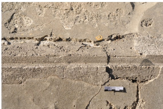
Figure 5: filling with hard mortar (cement?).
