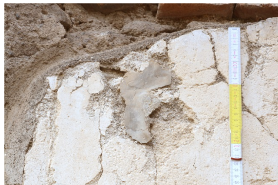
Figure 6: fillings mortar contains presumably plasticizer.
