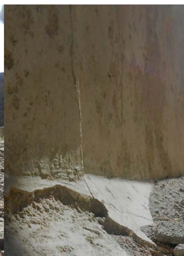
Fig 38 – more detail of Fig 37 where is evident the great attention to obtain a compacted and smooth surface to help the running out of the water.
