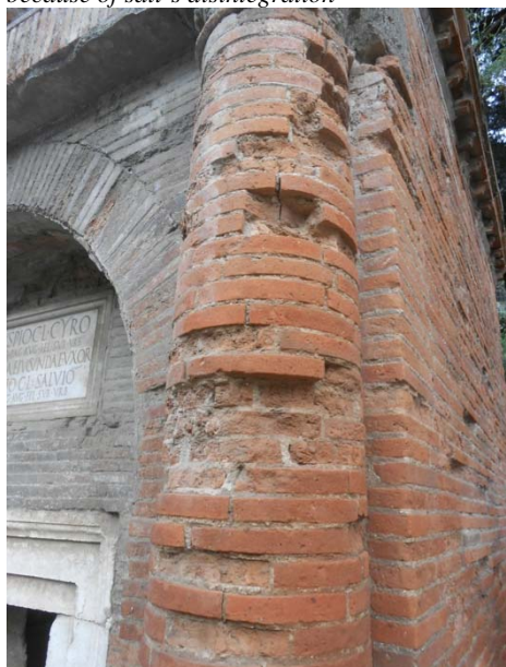
Fig 193 - Tomb 17ES, the decay slowly leads to the loss of the brick
