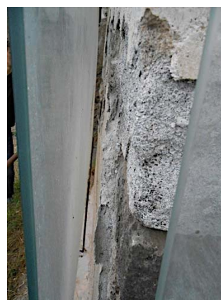
Fig 141 - Tomb FPND, detail of the modern glass protection which does not protect from the problems due to salt crystallization and mortar erosion.
