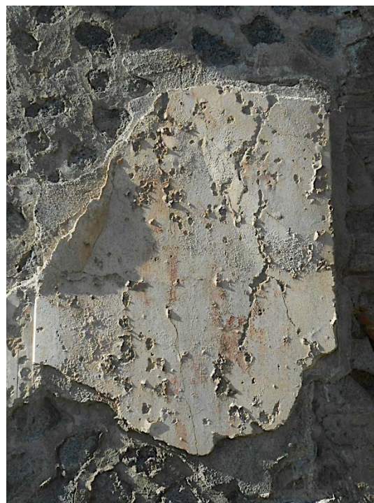
Fig 180 – Tomb 14EN, large portions of the external finishing layer of the stucco start to be pushed out from the surface.
