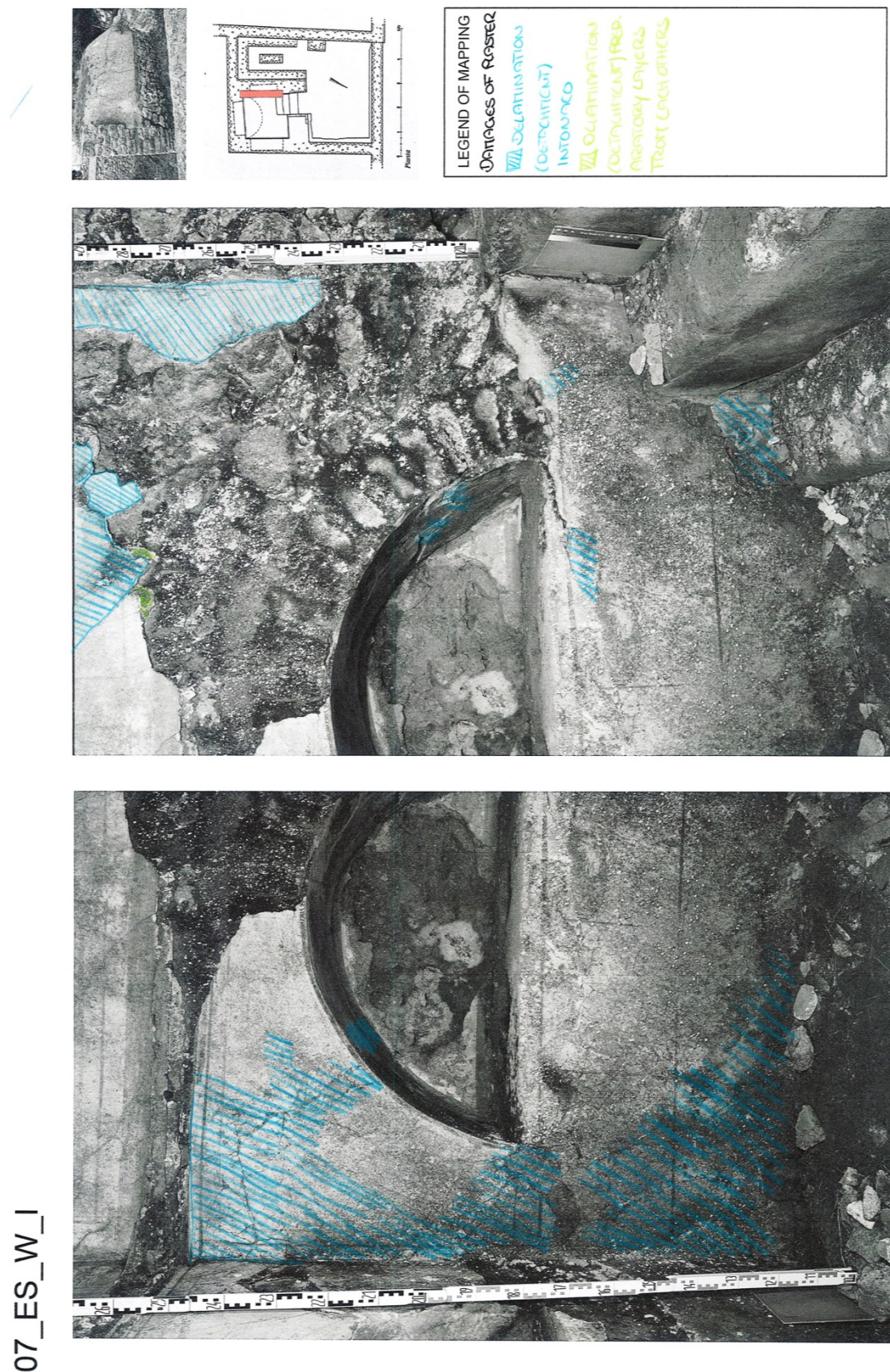
Figure 184: map 07_ES_W_I_1 of delamination (detachment) Intonaco from preparatory layers (blue) and delamination (detachment) preparatory layers from each other's (green).
