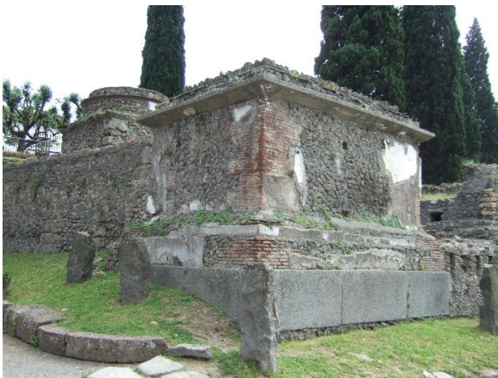
Fig 16 - Tomb 1 OS – general view, with volcanic stones for the basement and for the upper cornice, lava stones for the outer faces of the inner core structure and brick reinforcements on the corners.
