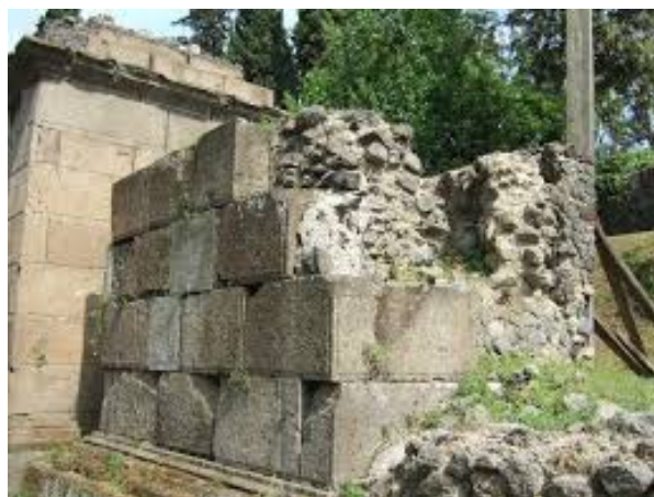
Fig 27 – Tomb 19OS, internal core in opus caementitium and external covering in stone blocks.
