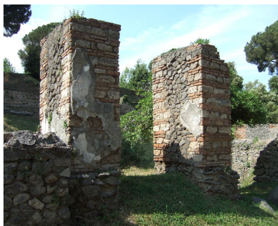
Fig 21 - Tomb 28EN - bricks as opus listatum in the pillars.
