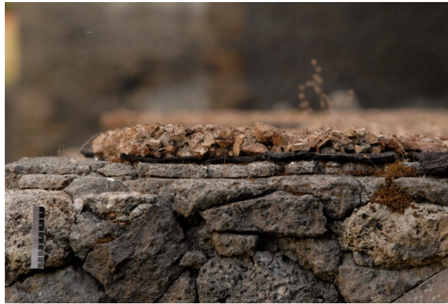
Figure 4: “modern waterproofing of original structure” at funerary monument 25_OS. Visible are layers of cement over an reconstructed masonry. Over the cement a layer of bitum and on top “cocciopesto”.
