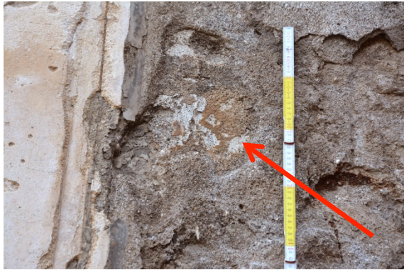
Figure 7: brown discoloration in missing parts of preparatory layers (red arrow).
