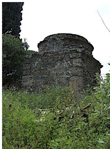
Fig 19 - Tomb 3OS - volcanic stone blocks used as reinforcement of the corners.
