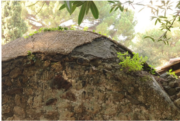
Figure 28: reconstructed roof with layers of cement, bitumen and “cocciopesto”.
