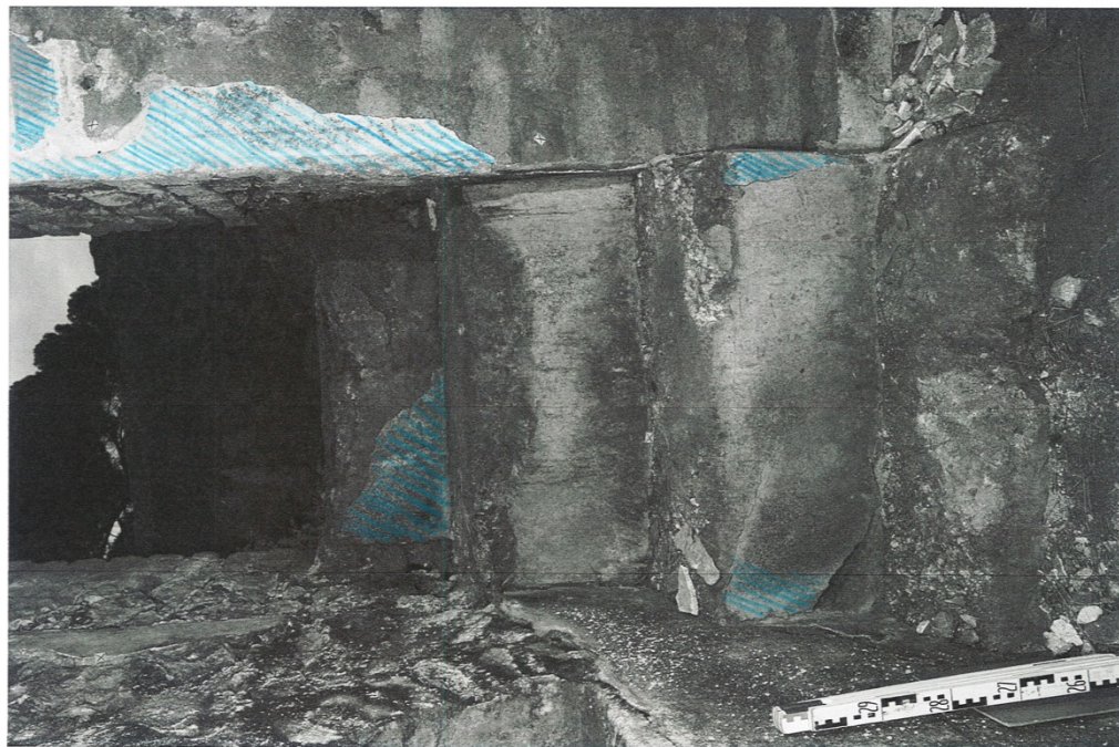
Figure 179: map 07_ES_N_I_1 of delamination (detachment) Intonaco from preparatory layers (blue) and delamination (detachment) preparatory layers from each other's (green).
