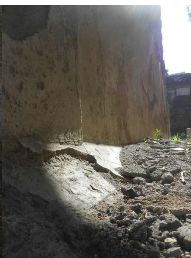
Fig 37 – another view of the same collector where the perfectly finished surface is evident.
