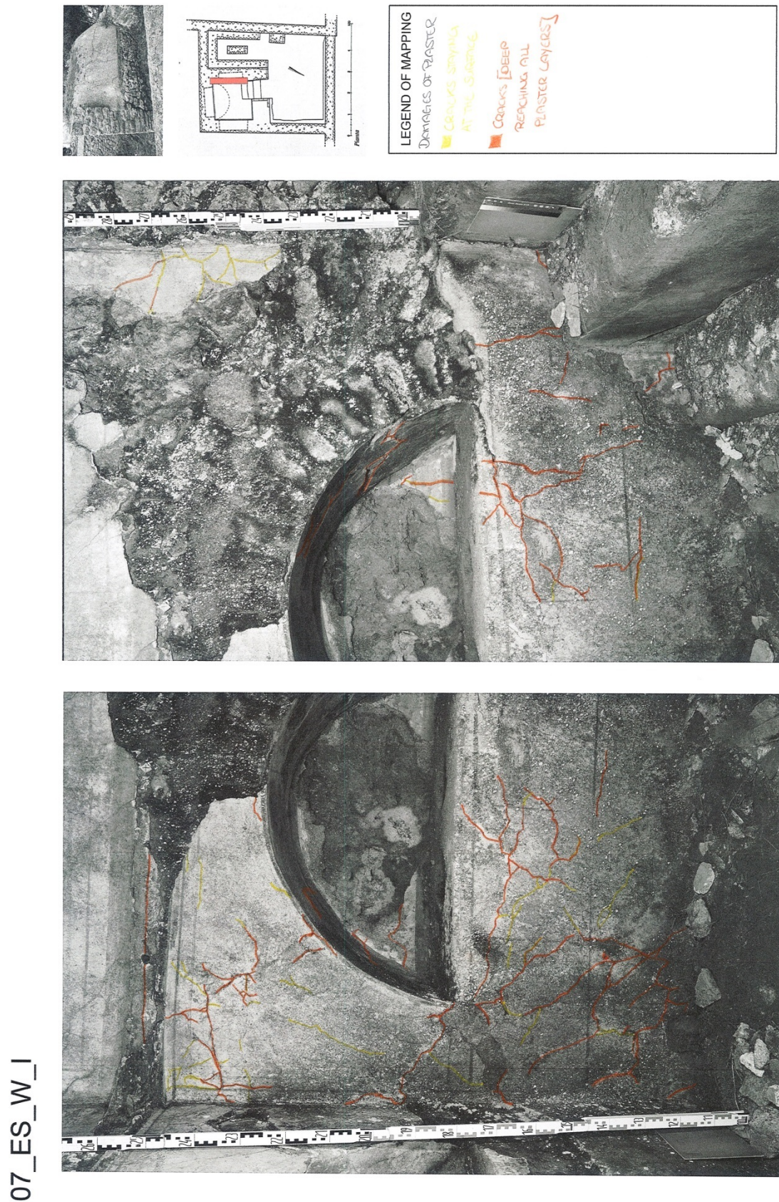
Figure 198: map 07_ES_W_I_1 of cracks.
