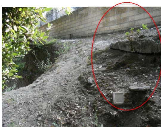
Fig 129 - North side of the pedestrian walkway wall. At the right of the image a phenomenon of erosion of the ground.
