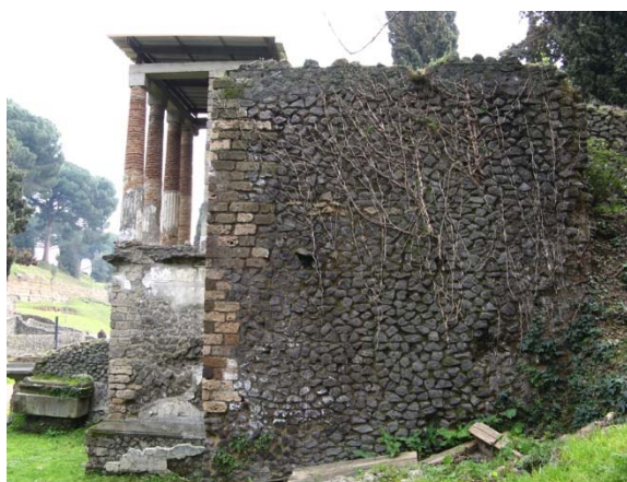
Fig 163 - 164 – Tombs 12EN and 15OS, more died climbing plants, pushing out the plasters in the right Fig. and over the surface which has totally lost the stucco covering.
