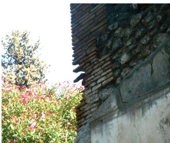
Fig 194 - Tomb 14EN., the loss of the single bricks can lead furtherly to structural problems, especially in the corners of the monuments
