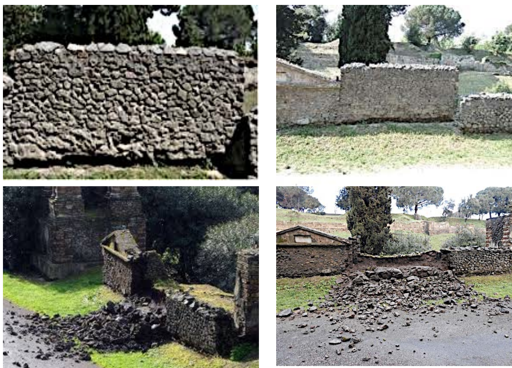
Fig 149- 150- 151- 152 - Tomb 24EN, the wall before and just after falling down, in March 2014. It is probable that the foundations have been slowly eroded by the rising damp and the rain.
