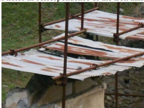
Fig 104 - Tomb FPN F, temporary roof in bad condition
