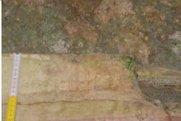
Figure 44: intense green infestation (picture number: 07_ES_W_I_BO_DSC_3173).
