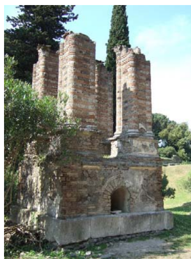
Fig 174 - Tomb 20EN, the foundations are exposed at the bottom of the front side.
