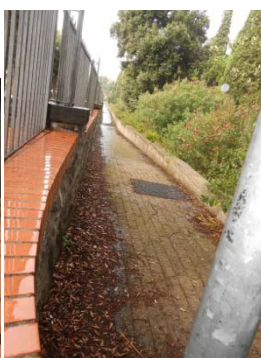
Fig 124 - view from the East of the slopes of the walkway, which run in two directions, both bringing the water towards the central part of the path, which corresponds (see next Fig.) to the upper area of the protective roofing which covers the “deposit” of statues and stone fragments (at the bottom of the ancient via di Porta Nocera)
