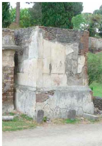
Fig 159 - Tomb 14EN in 2014. A big part of the left corner of the basement is gone.
