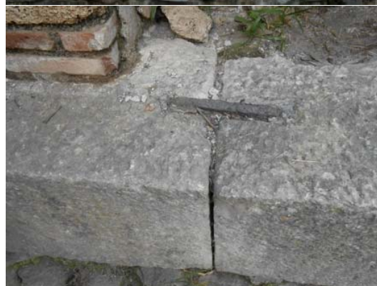
Fig 93 –Tomb 20EN, original clamp to hold together two stone blocks...
