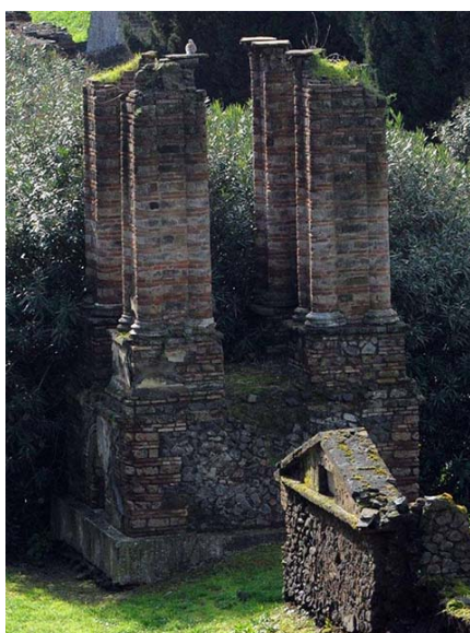
Fig 22 - Tomb 20EN – bricks as opus listatum in the columns.
