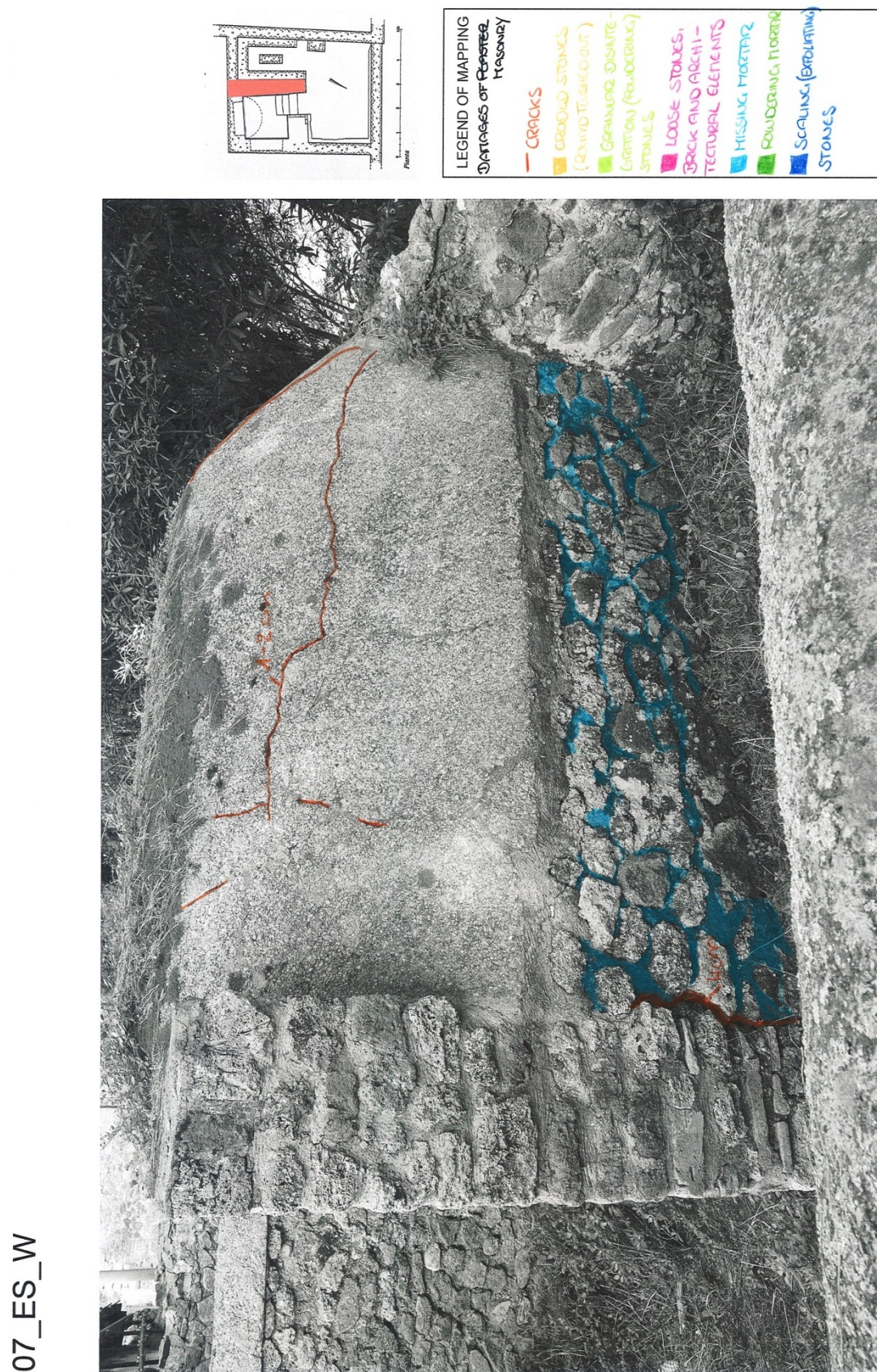
Figure 204: map 07_ES_W_E of masonry damages.
