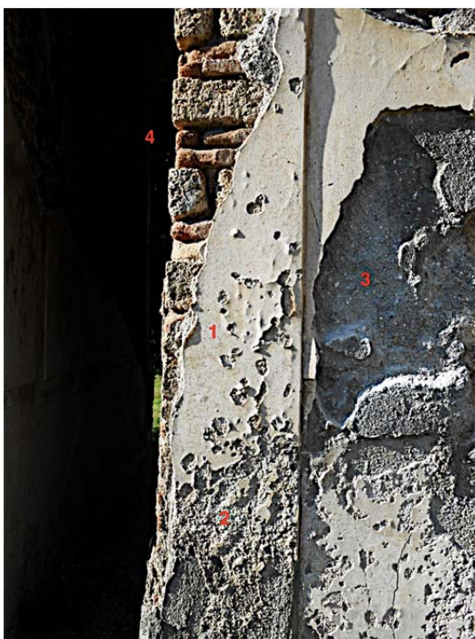
Fig 179 - Tomb 12EN, salt crystallization as:
