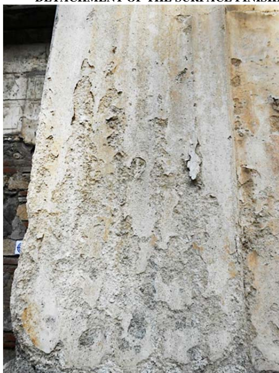
Fig 183 - Tomb 14EN surface of the "lesena" in stucco with a dramatic deterioration due to salts' efflorescences
