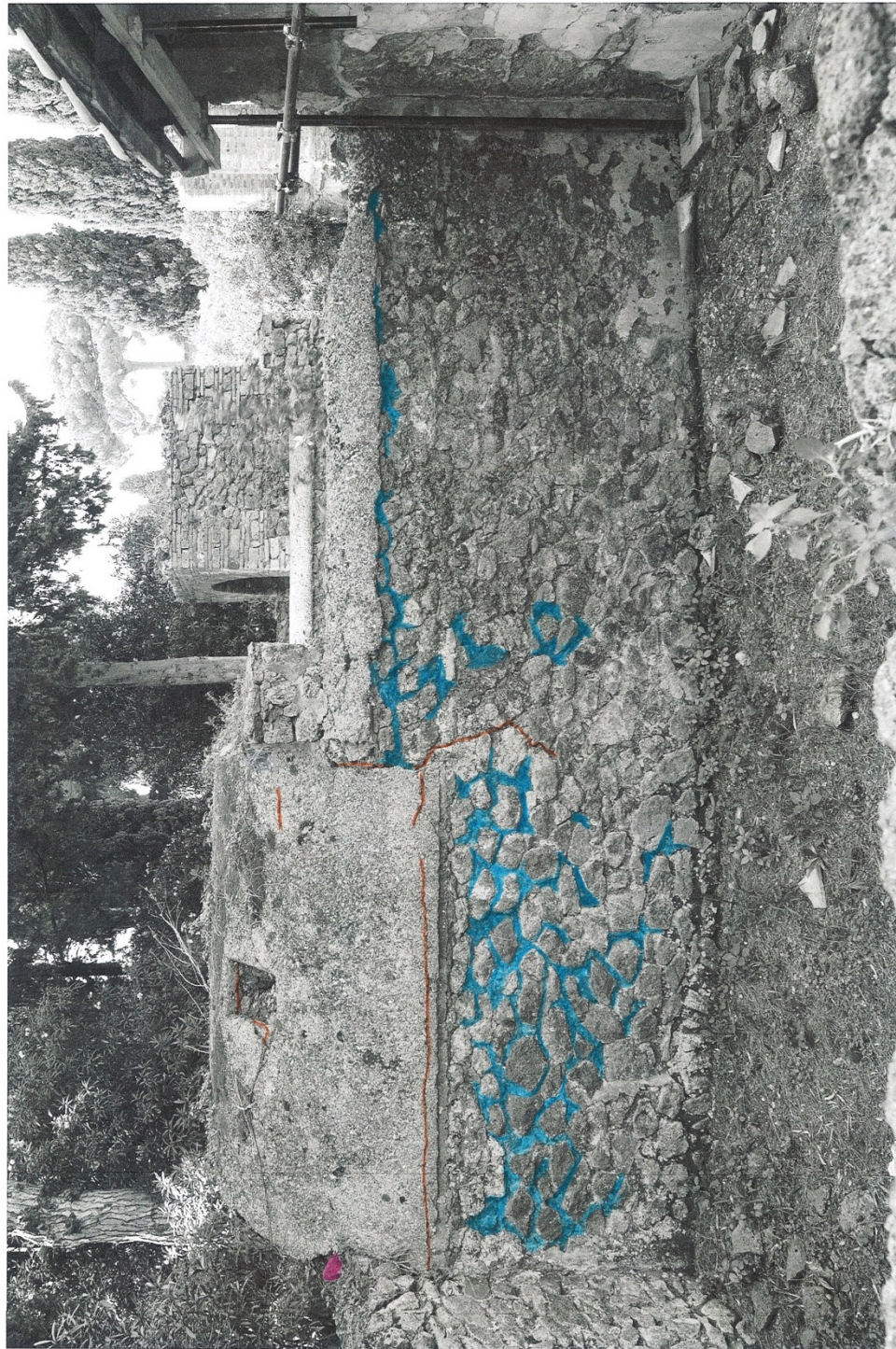
Figure 202: map 07_ES_E_E of masonry damages.
