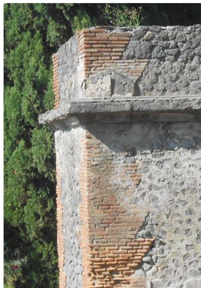
Fig 25 – detail of brick reinforcement in the corners of Tomb 10EN.
