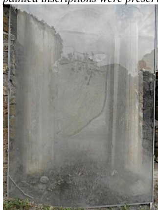
Fig 138 and 139 – Tomb 19ES – detail of the glass protection and its metal structure (left and right side). Due to the dust and humidity always present in the archaeological site, the glasses become dirty and opaque and the decoration is not visible anymore. Unfortunately it is not possible to clean the glasses, as they are not demountable.
