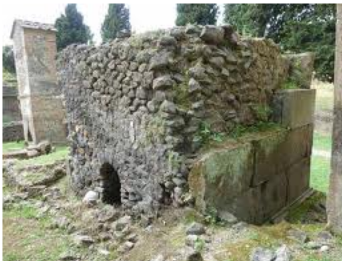
Fig 17 - Tomb 19OS – inner core in opus caementitium, back wall in with outer face in common lava stones (opus incertum) and more visible front faces in well-cut big volcanic stones (opus quadratum).
