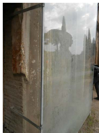
Fig 138 and 139 – Tomb 19ES – detail of the glass protection and its metal structure (left and right side). Due to the dust and humidity always present in the archaeological site, the glasses become dirty and opaque and the decoration is not visible anymore. Unfortunately it is not possible to clean the glasses, as they are not demountable.
