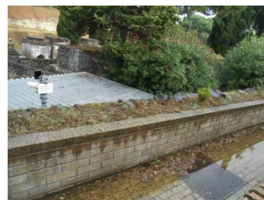
Fig 125 – the water stays in the depression of this area and slowly descends into the archaeological area through the provided water outputs.
