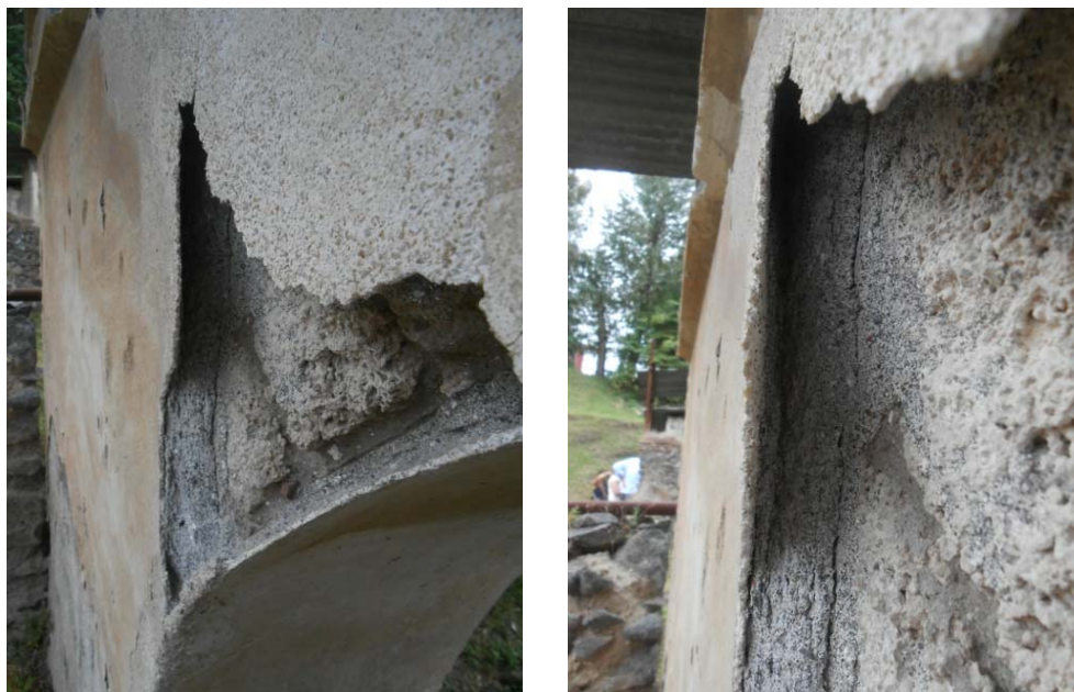
Fig 187e – Fig 187f - Tomb FPN.... erosion and powdering of the internal preparatory mortars, leaving the external finishing layer (more compact) totally unprotected
