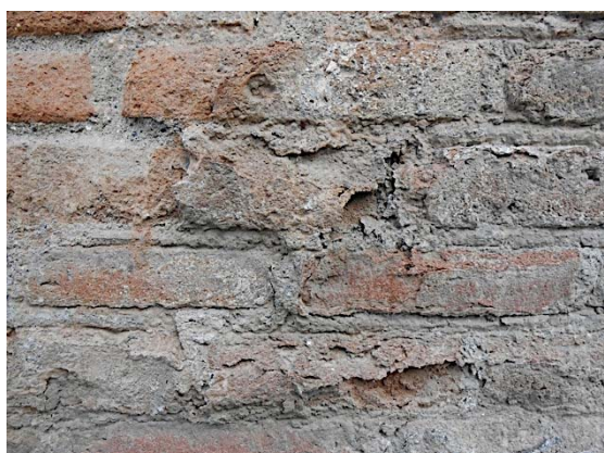
Fig 189 - Tomb 10EN, strong salt crystallization below the external surface of the bricks
