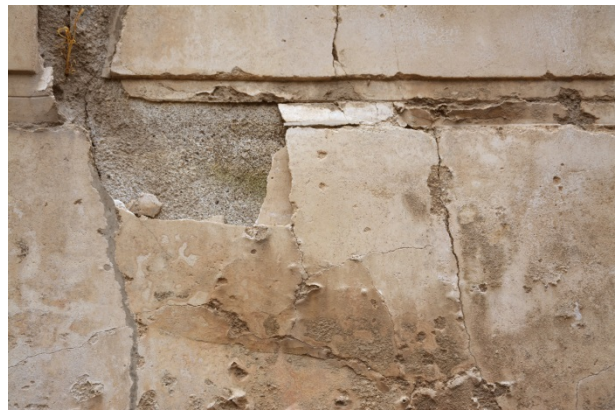
Figure 10: collapsing lacunae at 14_EN_S.
