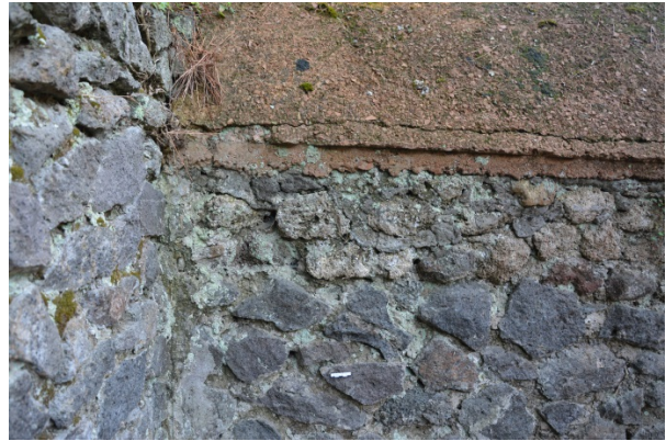
Figure 29: Fragments of original “cocciopesto” layers under a mounted reconstruction of “cocciopesto” roofing.
