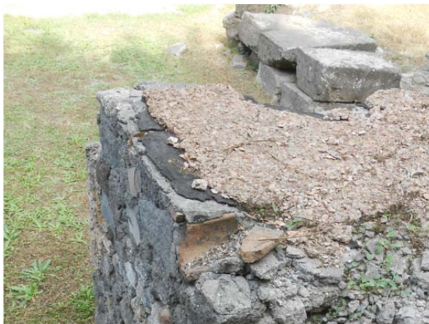
Fig 109, 110, 111 - Tomb 25OS General view and details of the modern impermeabilisation, which is repeated on many of the other tombs.
