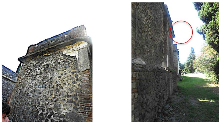
Fig 134 e 135 – back of the Tombs 6EN and 10EN – modern rain drains to collect the water from the top surface of the monument
