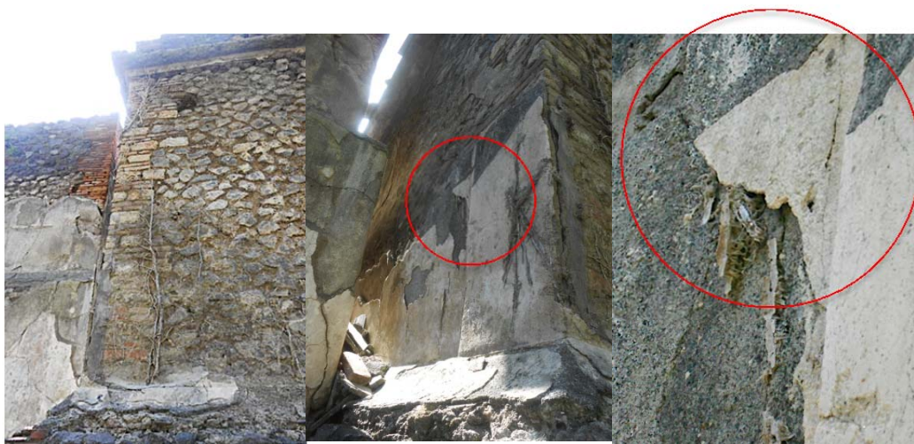
Fig 160 -161 - 162. - Back of Tomb 12EN. with long remains of climbing plants. In the detailed at the right, the roots are below a very unstable fragment of stucco, “pushing it out” from the surface.
