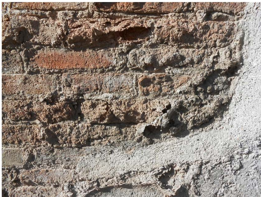
Fig 188 - Tomb 10EN, “explosion” of the external surface of the bricks due to salts crystallization
