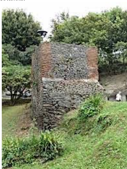
Fig 24 - Tomb 36EN – bricks as reinforcement of the corners.
