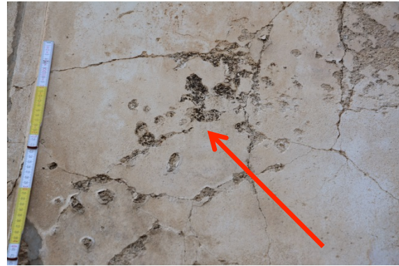
Figure 8: black discoloration in missing parts of Intonaco (red arrow).
