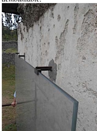
Fig 140 - Tomb FPND, detail of the modern glass protection with the metal elements to hold the glass in place.
