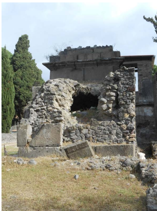
Fig 26 – Tomb 19OS – Internal core in opus caementitium and outer layer of stone blocks.
