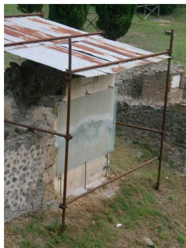
Fig 137 –Tomb FPND (ex Fondo Pacifico), glass protection on the South side.
