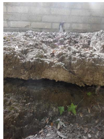
Fig 130 – detail of the previous Fig. The erosion of the ground is visibly linked to the water flow.
