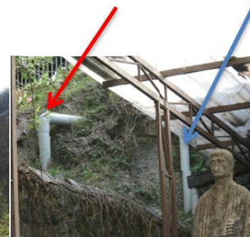
Fig 128 – the modern water collectors: from the pedestrian path in RED, and from the deposit roof in BLUE
