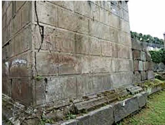
Fig 41 - Tomb 11OS, outer finishing with volcanic stone blocks.
