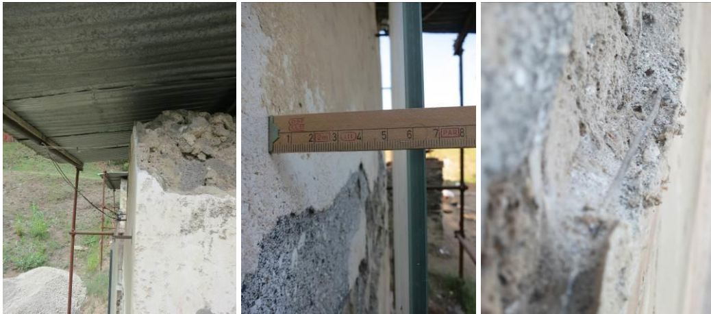
Figure 16: Detail of the gap between original wall and protective glass. The right picture shows the temperature sensor after one year. The sensor was placed on the edge of an open plaster. After one year the sensor is “buried” by down coming sand of airborne dust and the decomposing plaster above.
