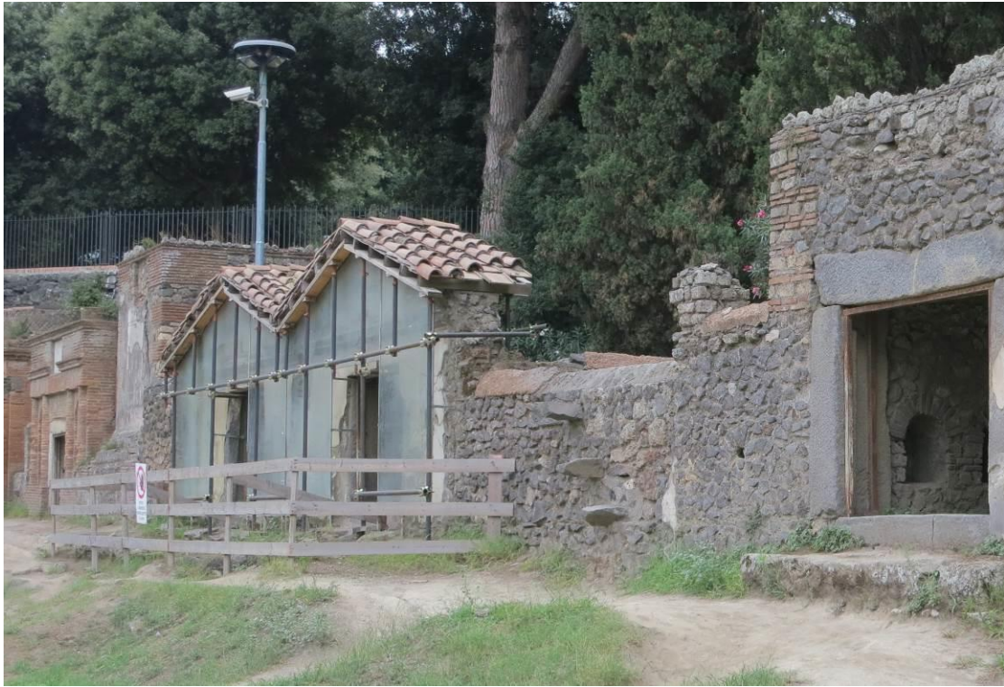
Figure 6: View from the street to the north side of tomb ES7 and ES9. The inner of the enclosure of ES7 is only accessible by the cantilever stone stairs. The front of ES 9 is protected by protective glass. Its wall roofing is supported by a scaffold.
