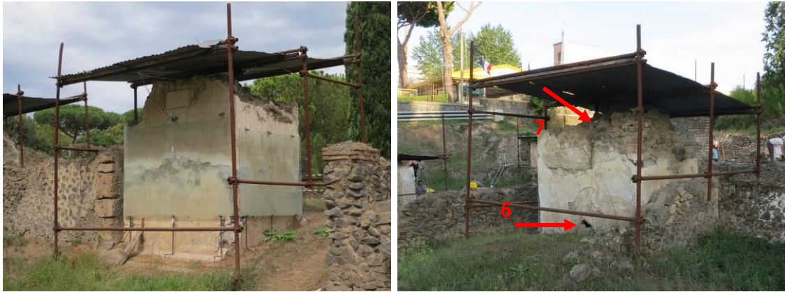
Figure 12: Tomb D-N-7 with view on the south and east side with protective glass (left picture) and view on the north and west side at the right picture. The arrows show the position of the data logger No 6 and 7.
