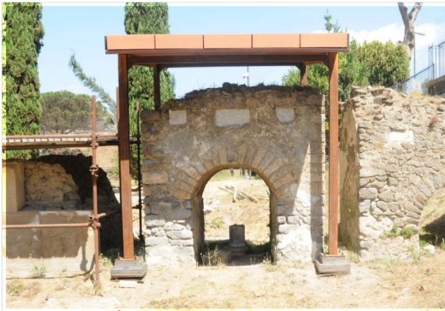
Fig.7: Prototype of the new covering roof developed by Fonti and Emmerling, TUM and installed on Tomb H of Via Nuceria in August 2017.
