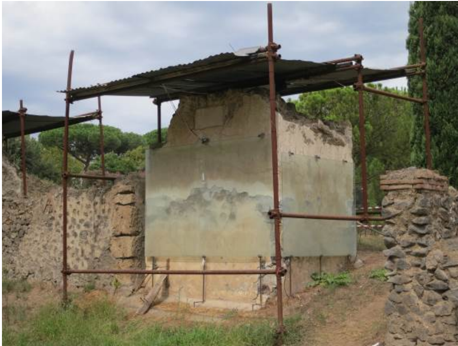
Fig. 2: South Façade of the Tomb D-N at the Via Nucerina Necropolis, Pompeii with a protective roof dating in the 1980s. A characteristic horizon of salt damages to the plaster can be observed.
