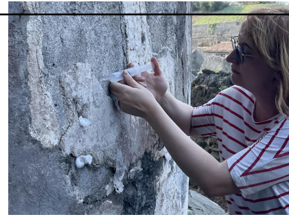
Prewetting before injection of the backfilling
